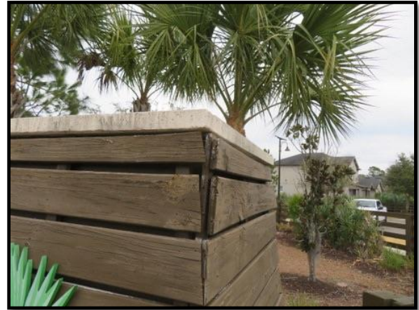
Figure 4 – Warped Boards.
